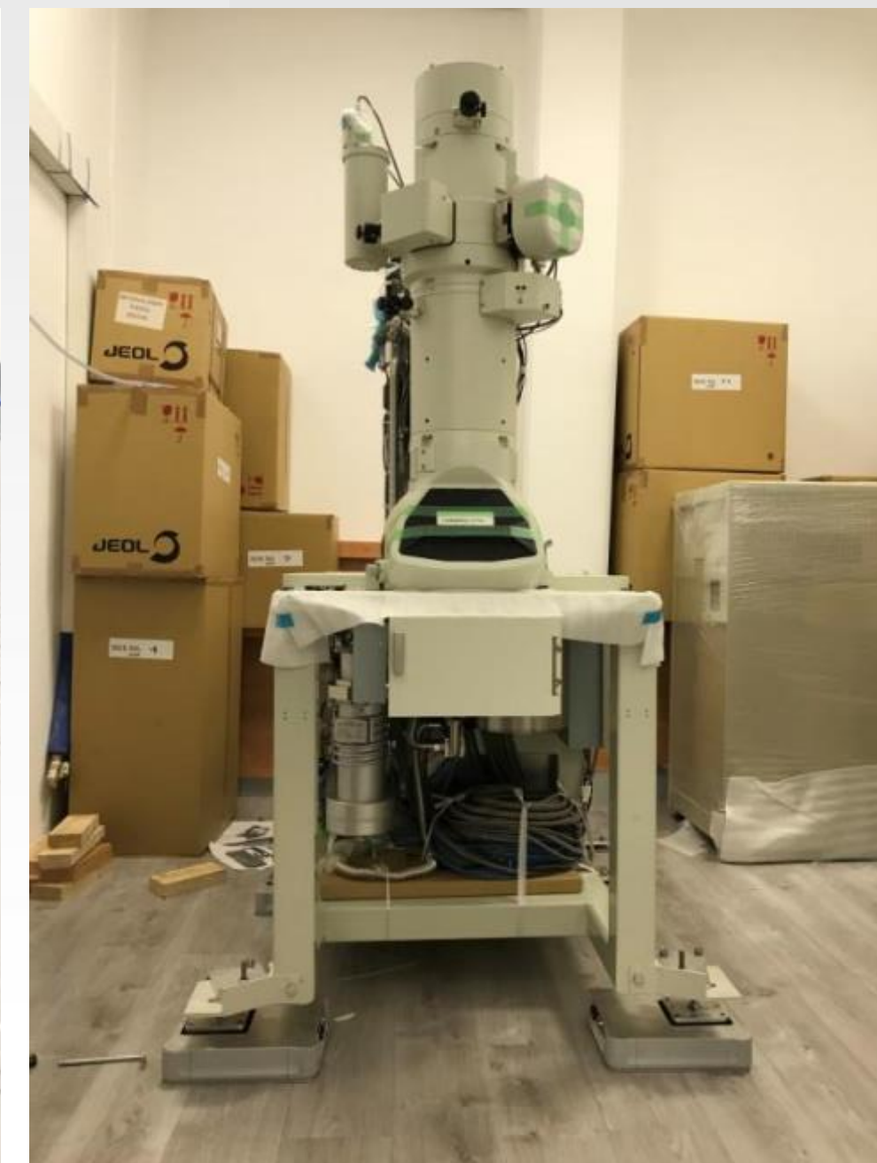
JEOL TEM Installed on a 4 th Floor
