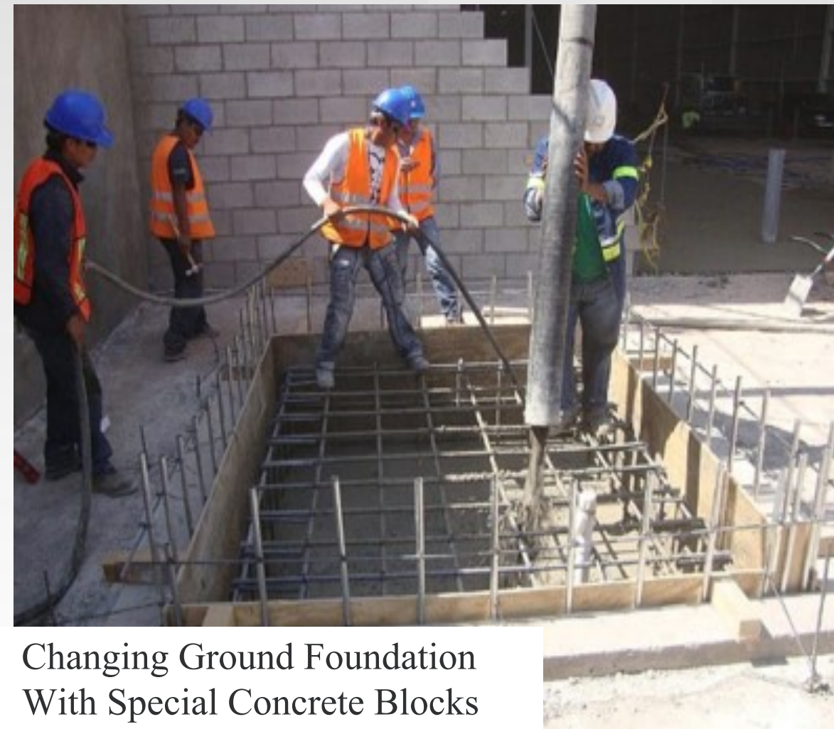
Passive Damping With Concrete Blocks
