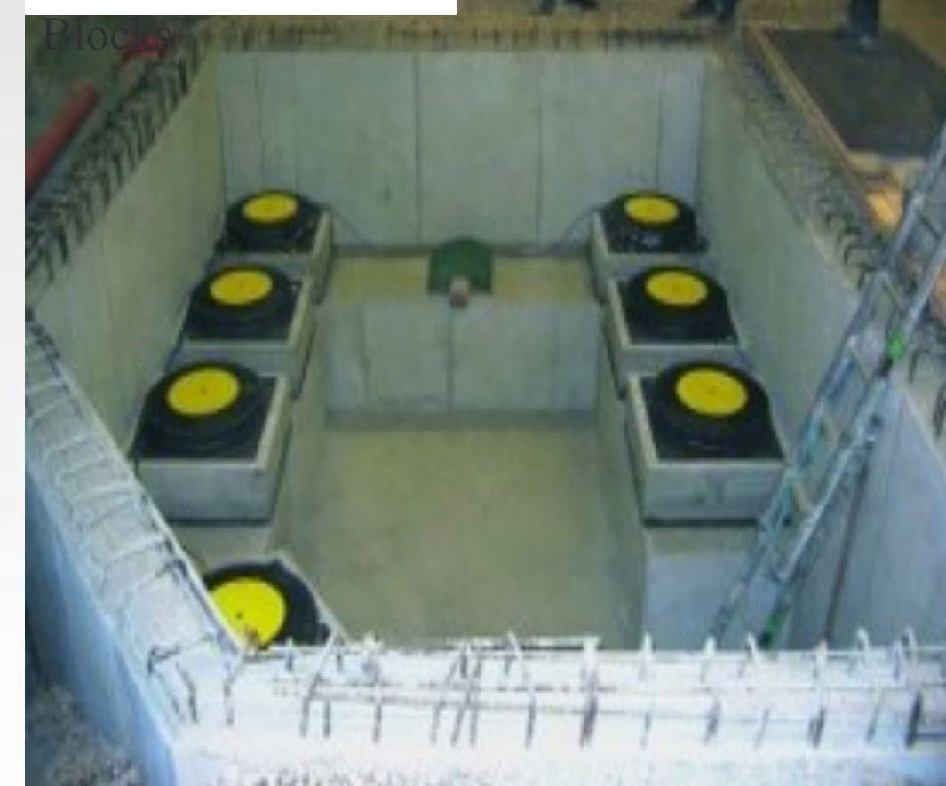
Passive Damping With Concrete Blocks
